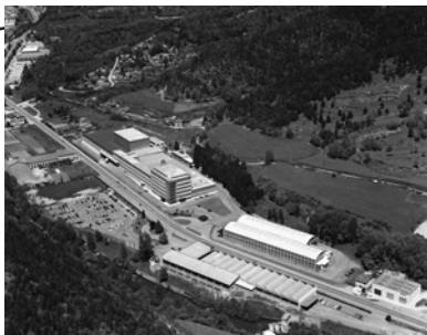
Ripoll Factory (Spain)
