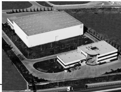
Logistics Center in Parets (Spain)
